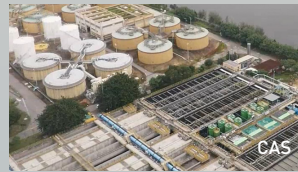
Sewage treatment area
