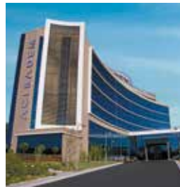
Acıbadem Eskişehir Hospital
